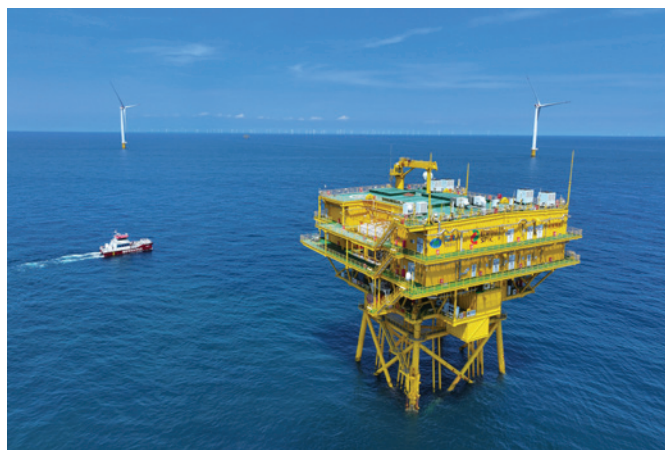
SPIC's offshore wind farm in Guangdong will supply renewable electricity to the BASF Zhanjiang Verbund site.
