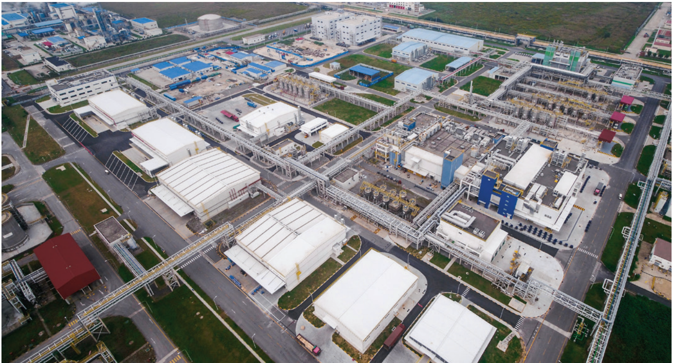
BASF Shanghai Caojing site; BASF Shanghai Coatings Minhang and Caojing sites, and BASF Coatings' resin plant in Caojing, Shanghai, realized 100% renewable energy usage across its operations in 2023.
